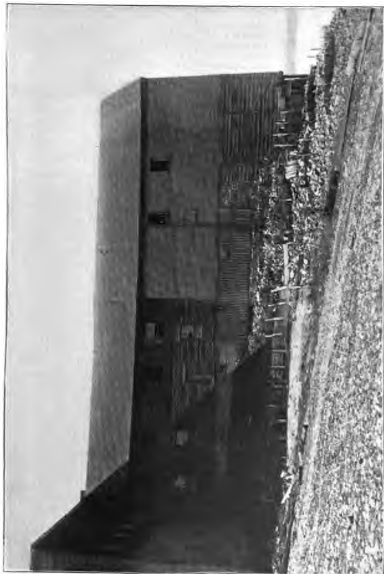
AUDUBON'S MILL AT HENDERSON, KENTUCKY.
